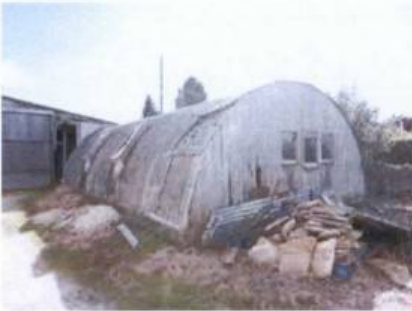
Existing barn structure - north yard
