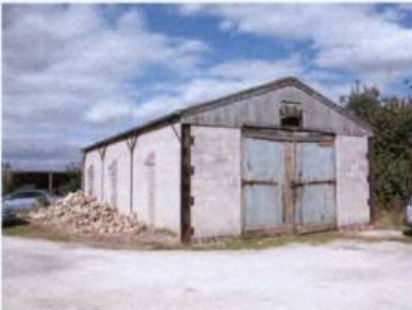
Existing barn structure - north yard
