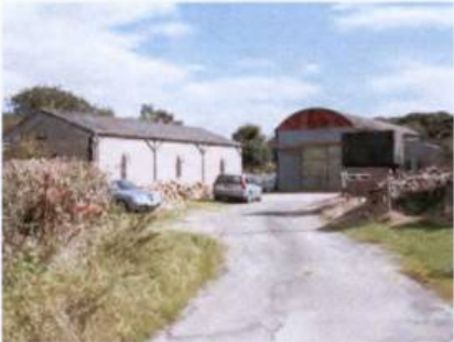
View to north yard from Chapel Lane
